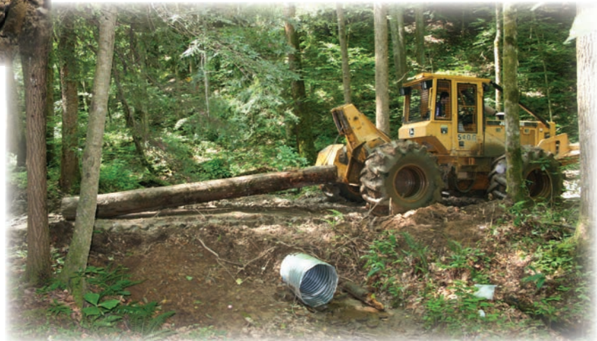
Figure 2 (right): Kentucky BMPs require the use of proper stream and channel crossing. This could include hard bottom crossings or the use of elevated crossing like the culvert shown above.
